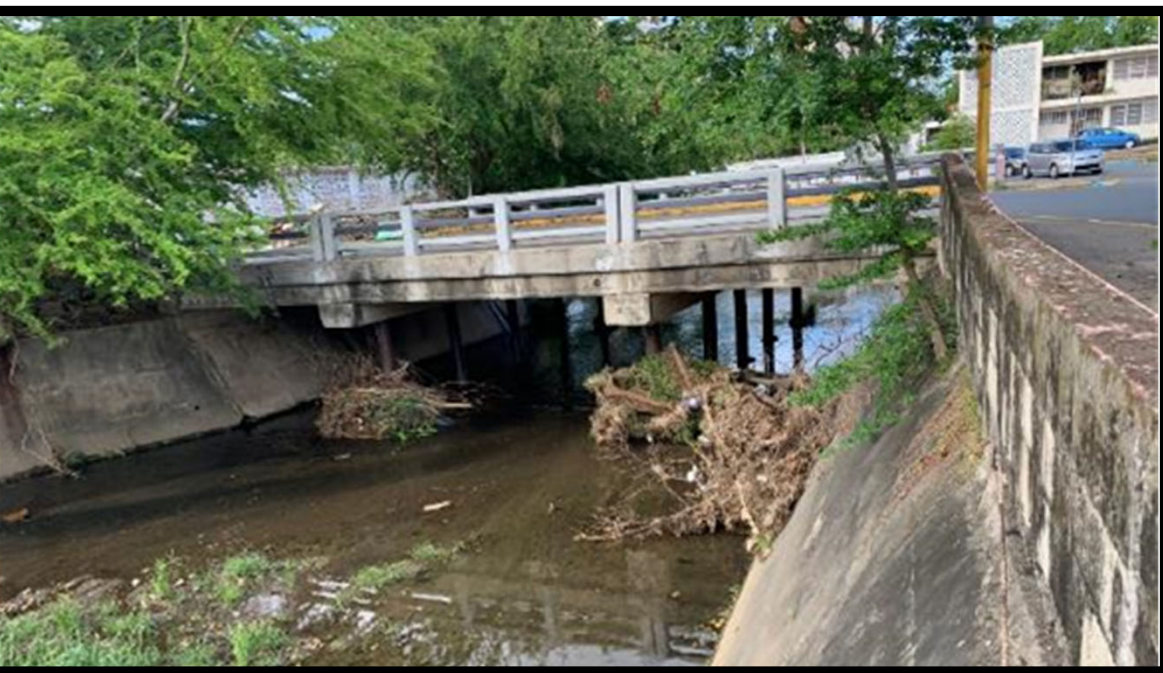
Figure 2: Image of existing conditions of Andalucia bridge.
