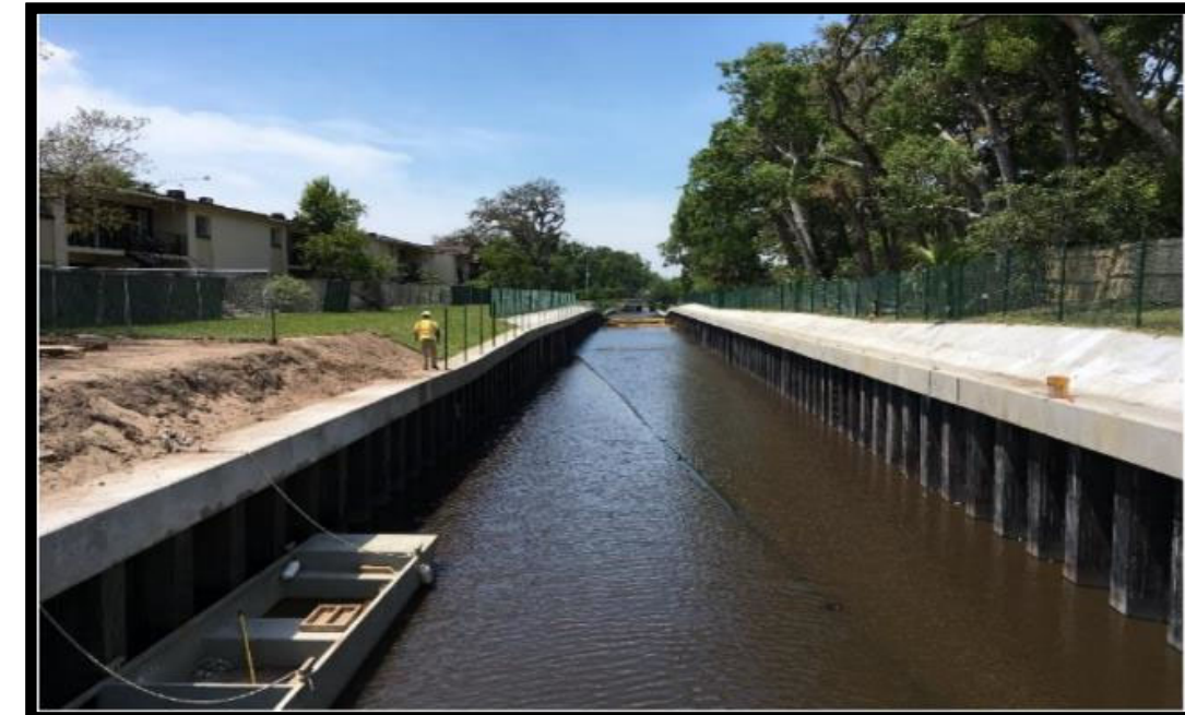
Figure 3: Example of actual construction similar to what the Josefin and Doña Ana Channels will look like upon completion.
