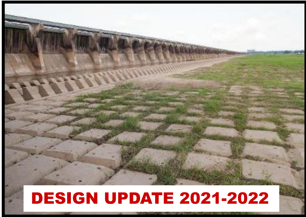
Articulated Concrete Block Mattress Channel Bottom
